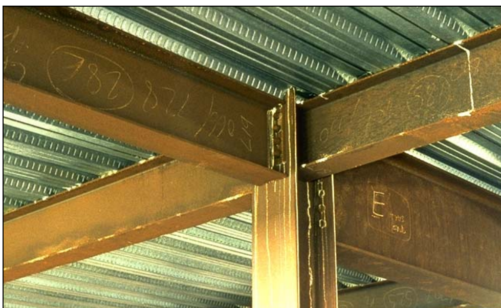
Figure 1-2 View of unprotected steel structure
