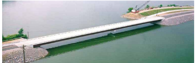
Martin's Creek Bridge in Tennessee
