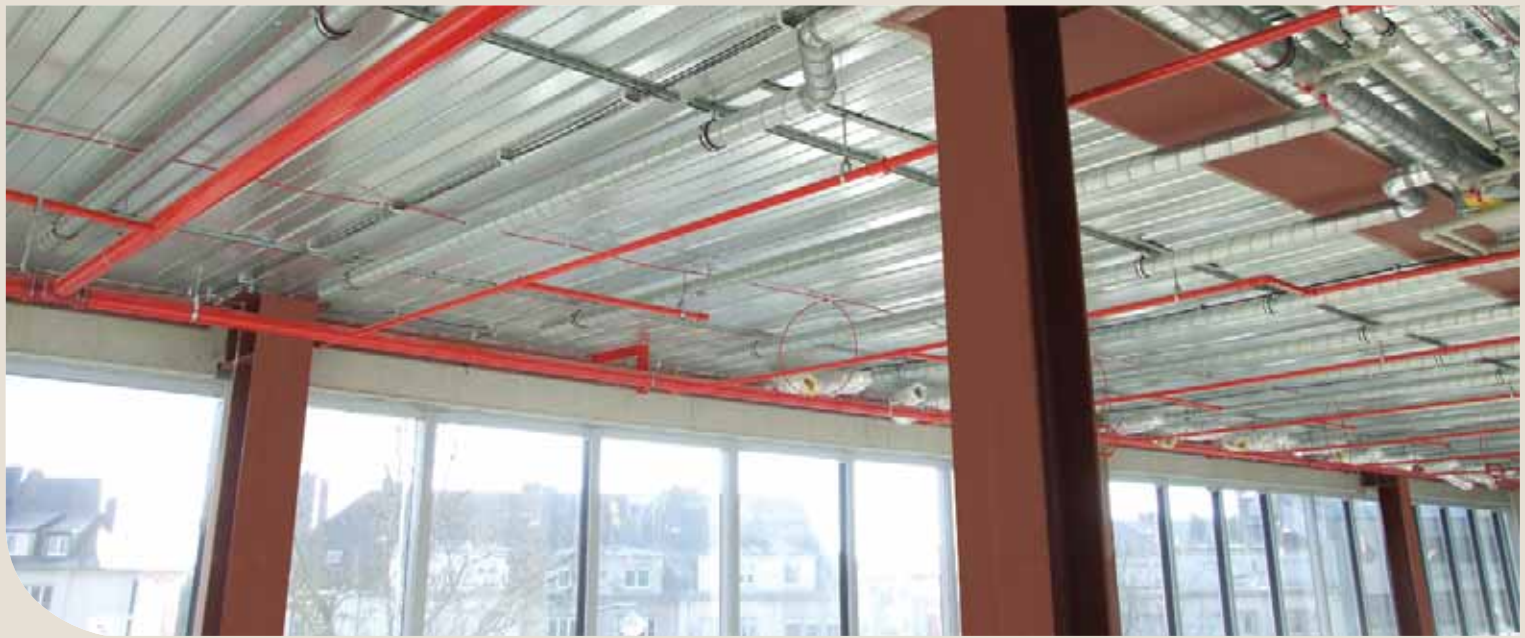
Figure 1: Slim-Floor Construction with Cofradal slab
