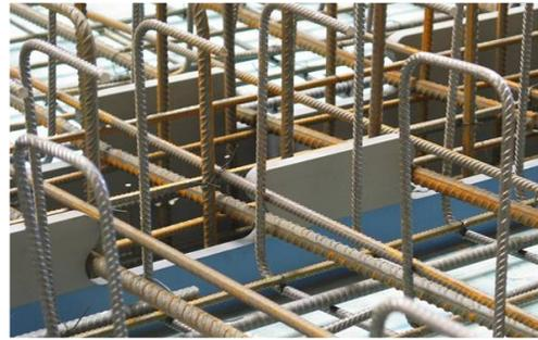
Fig. 5 – Reinforcement for prefabricated concrete plate
