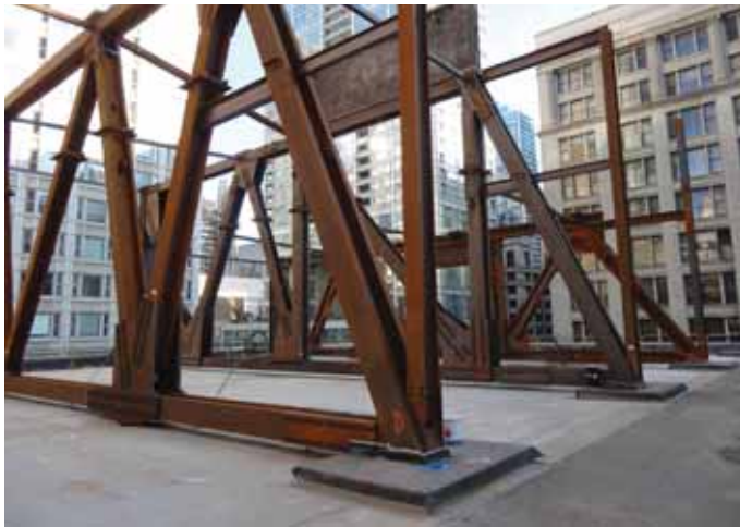
A913 Grade 65 sections used in transfer trusses
