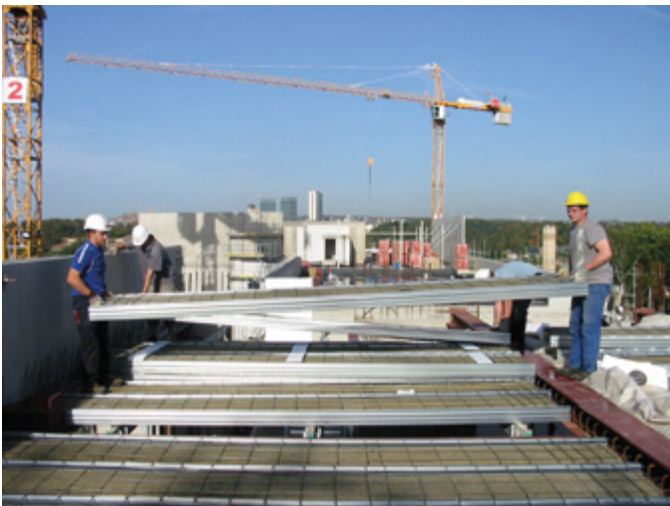
Installation of Cofradal® 200
