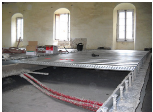
Installation within rehabilitation project - Cofraplus® 60
