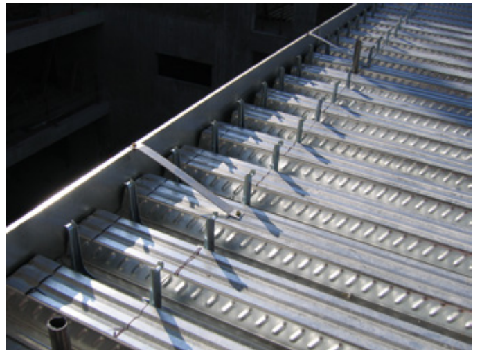
Edge trim with restraint strap and nailed shear studs
