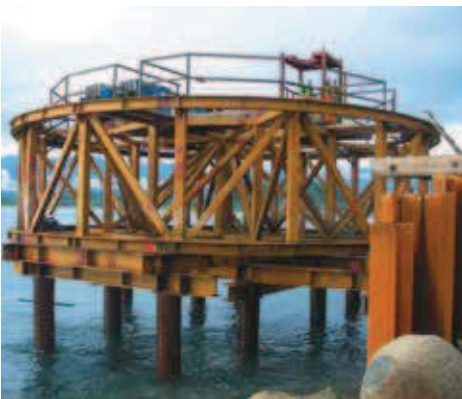
1. Installation of template
