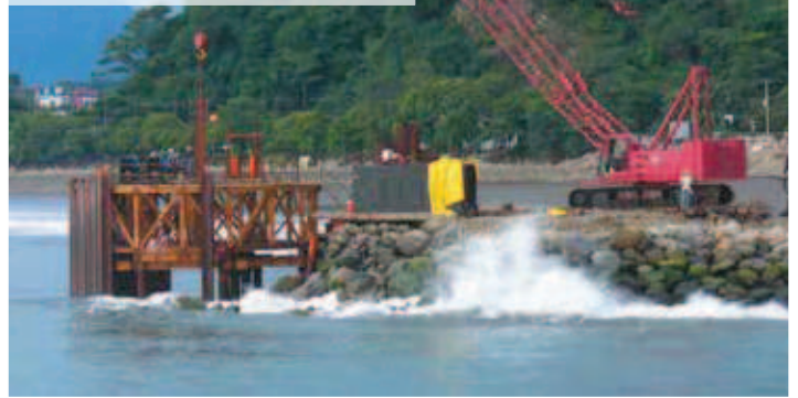
Marina breakwater, Costa Rica
