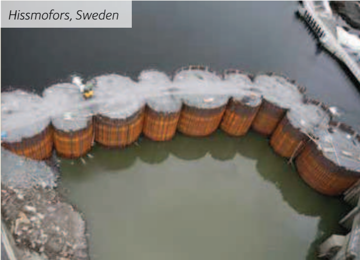
Circular cells with 35^\circ junction piles and one or two connecting arcs.
