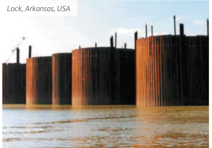
Diaphragm cells with 120^\circ junction piles.
