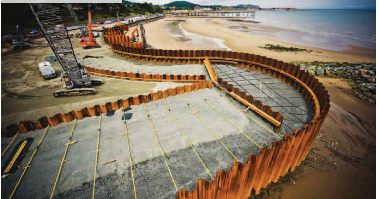
Costal defense project, Colwyn Bay, UK
