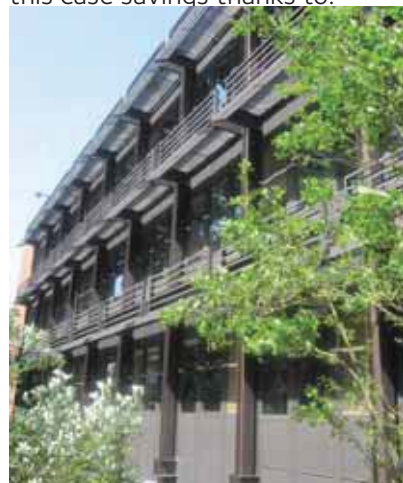
Office Building, Esch/Alzette (L)
