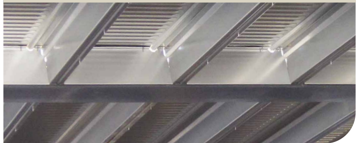
ABB: Detail Slim-Floor-System
