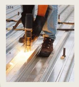
Studs welded through the metal deck on site Comparison between different steel grades for a non composite floor system Comparison between different steel grades for a composite floor system
