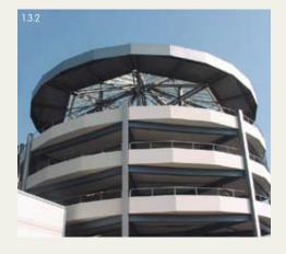
When designing the façade of a multistorey car park, a major part of the outside walls should remain open (pic. 1.3.2).
