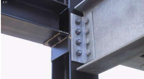
The steel bearing structure consists of vertical columns and horizontal beams, usually connected by bolting (pic. 3.1.1). The horizontal forces due to wind and breaking of cars are transferred horizontally through the floor slabs to the vertical wind bracings or shear walls (e.g. stiff staircases).
