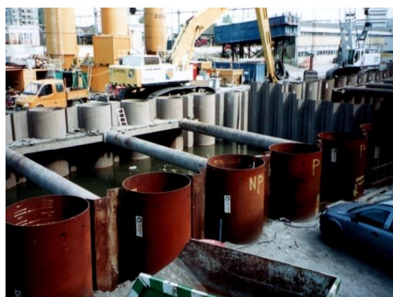
Figure 4 - Left: Installation of infill sheeting; Right: CombiWall with waling for the new central railway and metro station in Rotterdam (2008).
