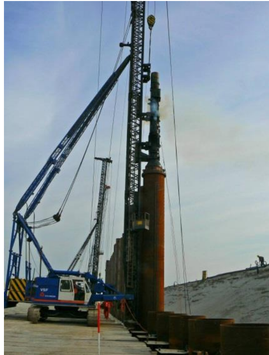
Figure 7 - New quay wall in harbour extension Rotterdam into the North Sea.
