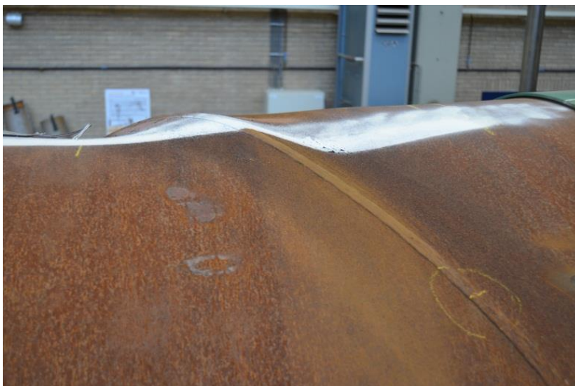
Figure 73 - Photo of the only observed buckle close to a spiral weld.
