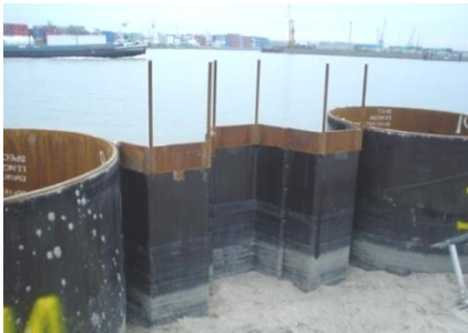
Figure 2 - Schematic and photo of a CombiWall (combined wall of tubes and infill sheeting connected with welded slots to the tube).
