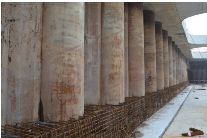
Figure 44 - Inside of building pit during construction with accessible combined walls.
