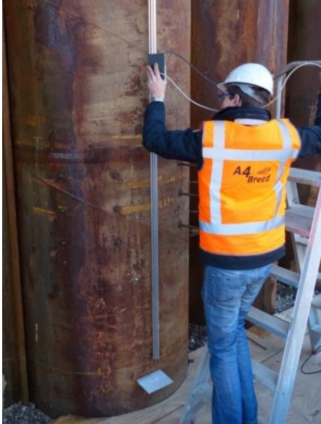
Figure 45 - Measuring of imperfections in building pit.
