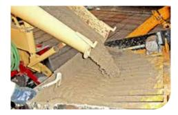
The concrete mix design should show a stable gradual curve with a maximum aggregate size of 16 or 22 mm in some areas.
