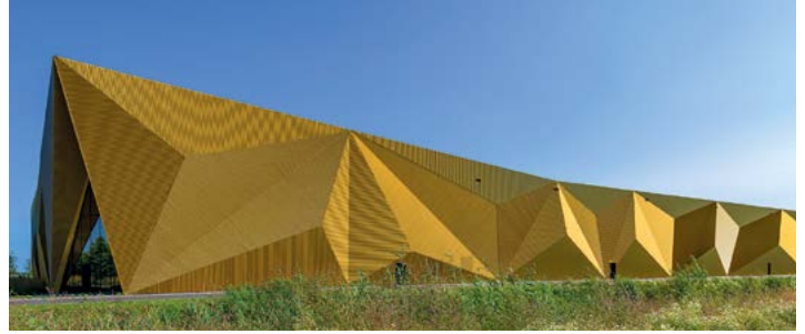
New Royal Dutch Mint building in Houten, the Netherlands – Architect: WILMA WASTIAU Cladded with Granite® Silky Shine Gold – profiles
