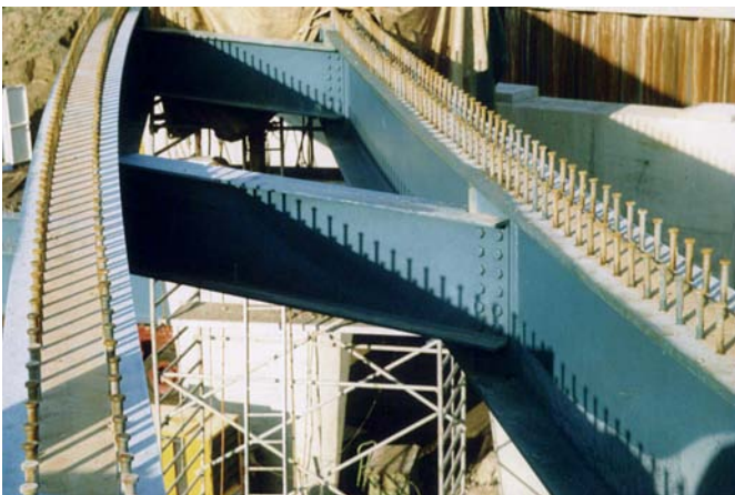
Fig. 16: Execution of detail of U-cross-beam bolted to a stiffening plate; left: practical example during construction; right: execution with drainage openings for galvanising
