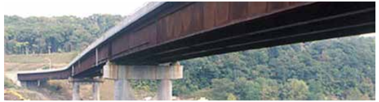
Ford City Bridge in Pennsylvania
