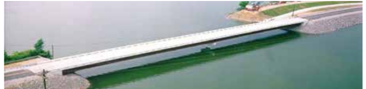
Martin's Creek Bridge in Tennessee
