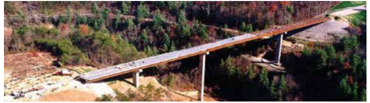
Clear Fork Creek Bridge in Tennessee
