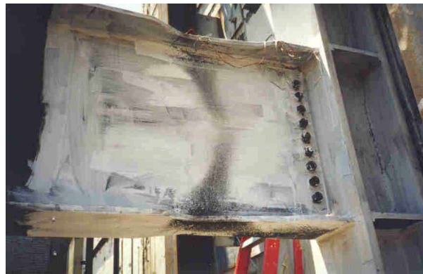
Figure 7. Reduced Beam Section (RBS) after testing
