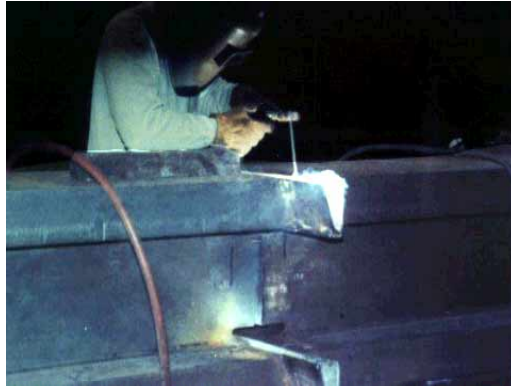
Figure 2. CJP butt-welding of ‘Jumbo’ shapes W14x730 (5 in. flange)
