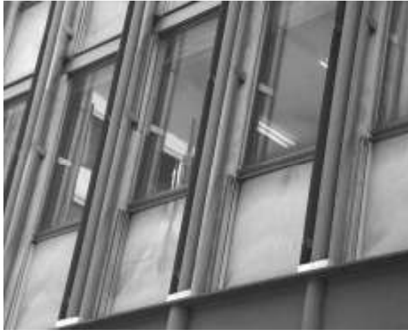
Figure 11 - Example of external columns protected by deflectors
