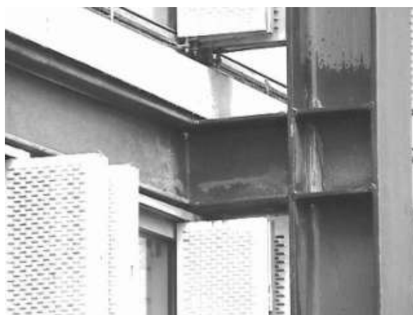
Figure 12 - Picture of external members
