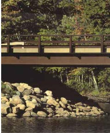
Questions also have been raised regarding the effect of acid rain on the corrosion resistance of uncoated weathering steel. Research conducted by ArcelorMittal USA laboratory indicates the effect of acid rain can be ignored. Wet deposition of sulfur dioxide, as in acid rain, actually has a beneficial effect on weathering steel because the acid rain washes away dry deposits that may increase corrosion.
