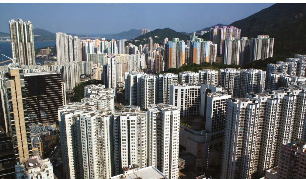
Figure 2. In order to maximize the internal, usable space, developers in Hong Kong could be motivated to simply “extrude” the floor plan, as protruding building features, such as balconies, can count against the total allowable floor area for a building site. © WING (cc by-sa)
