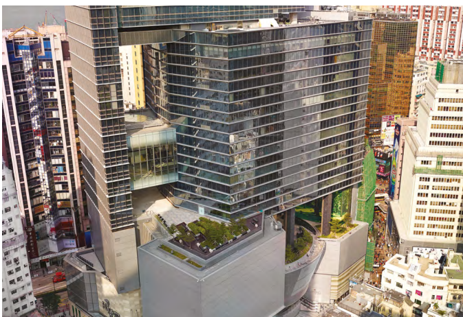
Figure 3. Hysan Place, Hong Kong took advantage of GFA exemptions by incorporating green features into the design. © Kohn Pedersen Fox Associates
