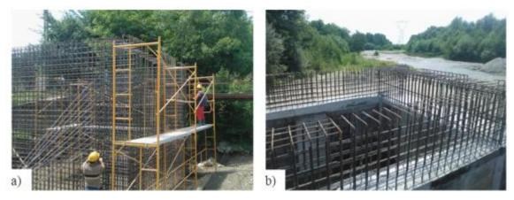
Figure 53 - Site photo of the abutment reinforcement (a), Site photo of the abutment (b)
