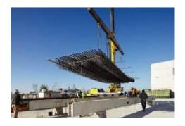
Figure 13 - Lifting of reinforcement-cage
