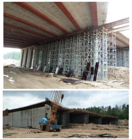
Finally reinforcement of girders and crossbeams was realised and realisation of superstructure could follow according to initially assumed design scheme:
