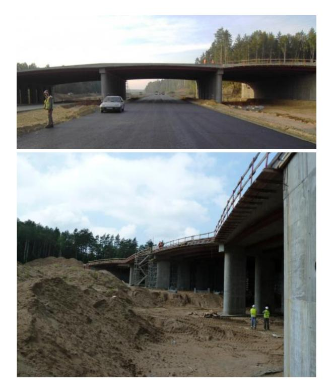
The next steps were to make embankments behind abutments, side concrete elements and soil on the superstructure.
