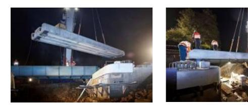
Figure 24 - Lifting of pedestrian bridge
