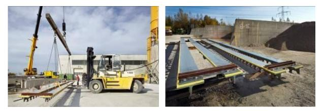
Figure 17 - Transport of external sections
