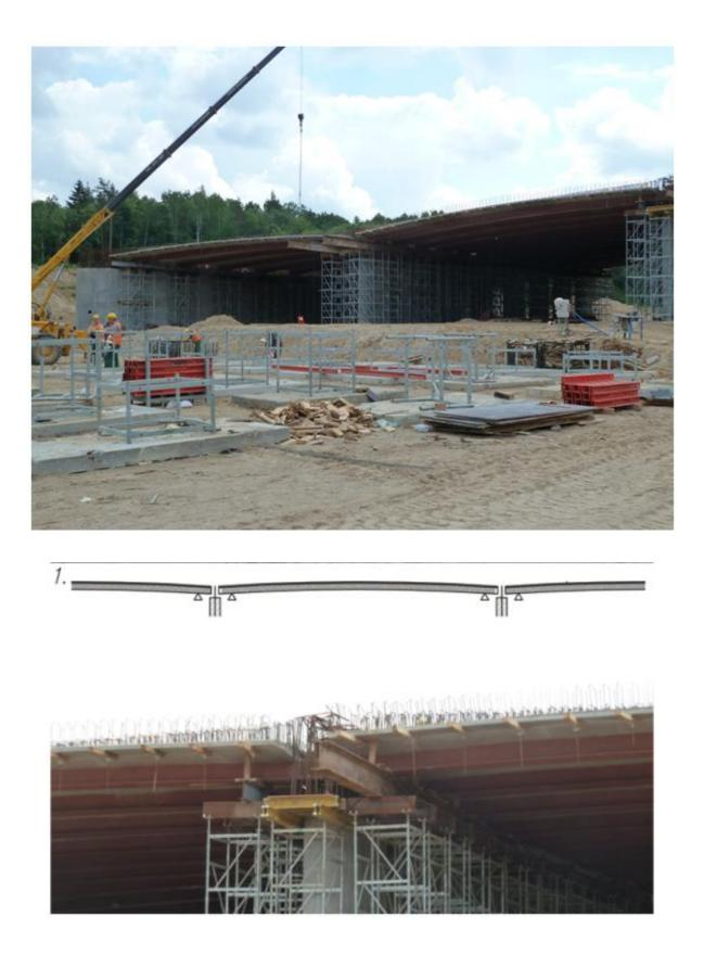
The view from the bottom of the bridge (picture below) presents prefabricated girders of line 2 on temporary supports and realised structure of line 1:
