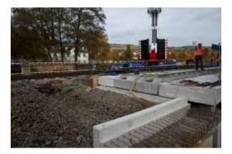
Figure 27 - Bridge(s) after mounting
