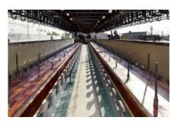
Figure 14 - Rebar-cage above formwork
