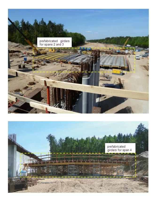
Girders have been realised and they were shifted by crane to their final positions on temporary supports next to pillars and abutments. Temporary supports were necessary to realise scaffolding for crossbeam proper way also.
