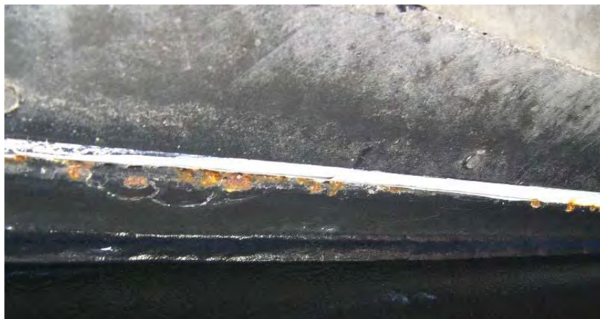
Figure 5-15. Corrosion in the interface steel-concrete [33].
