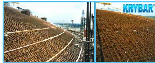
Figure 17 – Reinforcing steel for concrete reinforcement of LNG storage
