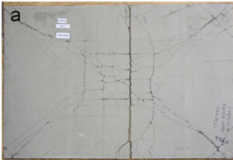
Tensile failure of reinforcement
